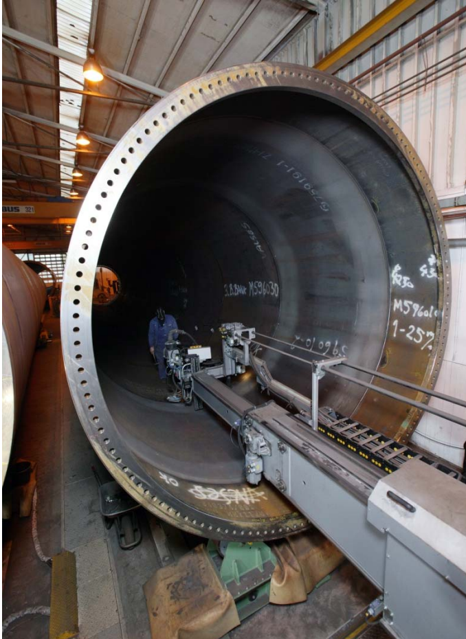
Internal welding with Telbo™
